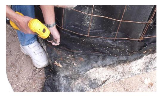
Figure 5. Screwing the Base of the Cage to the Pallet
